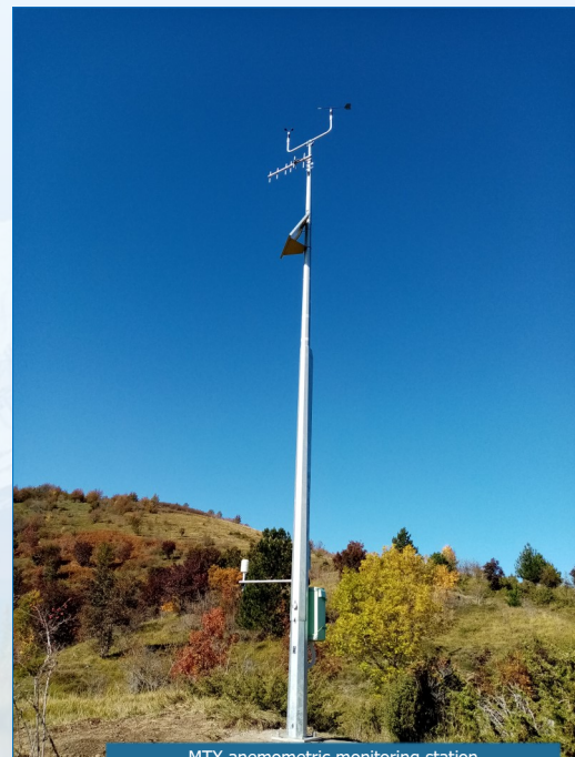
MTX anemometric monitoring station
