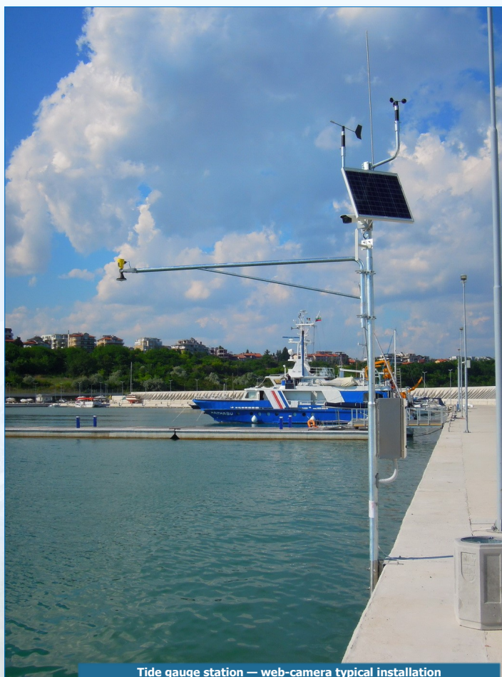
Tide gauge station — web-camera typical installation
